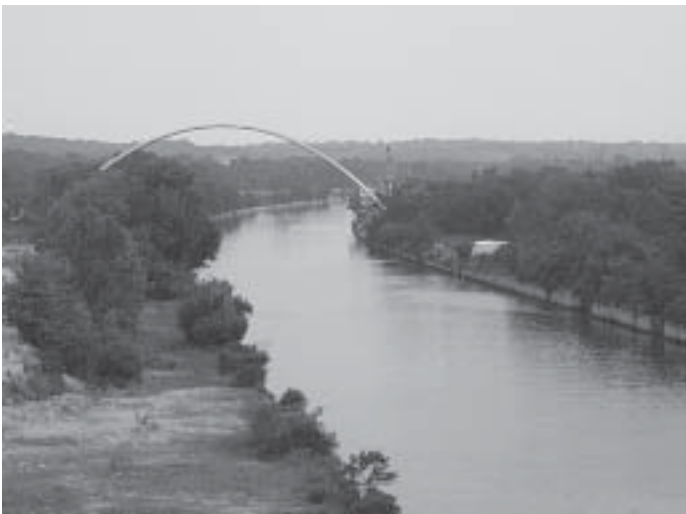
The electric barrier is located in the Chicago Sanitary and Ship Canal near Romeoville, Illinois. (The arch over the canal is a gas pipeline and is not related to the barrier.)
