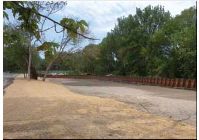
The West Branch Grand Calumet River in Hammond, Indiana has undergone remediation through the Great Lakes Legacy Act.
