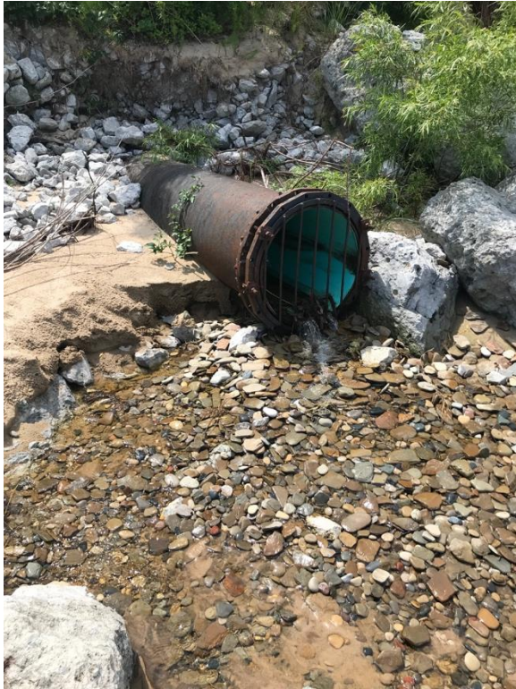
Figure 1 Stormwater outfall at Stop 24; discharges consistently in both wet and dry weather directly onto beach.
