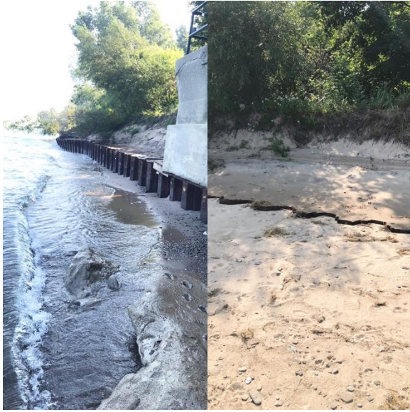
Figure 2 Evidence of beach erosion at Stop 25. Photo on left taken September 2, 2019; photo on right taken July 25, 2019. Prior to July 25 th sampling date, seawall was completely covered by sand. Sand height reduced by >30 cm.
